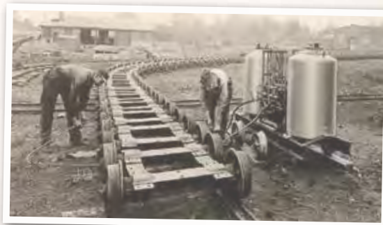
COAL CAR LUBRICATION SYSTEM
